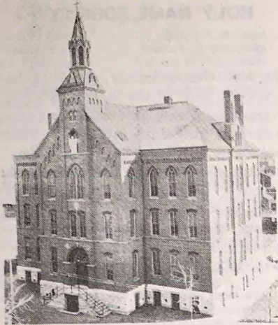
Old St. Francis School Building
